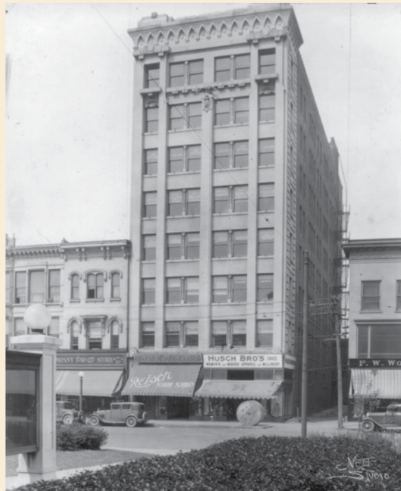
Reisch Building, Springfield, Ill. (1914-1920)
