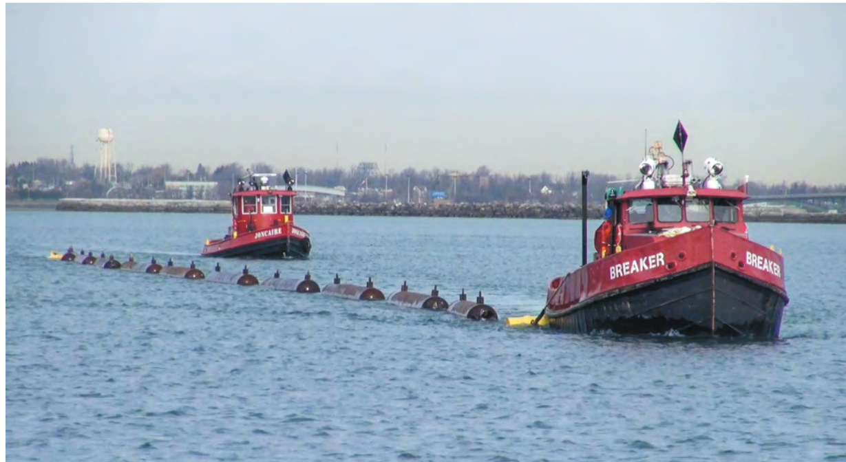
Niagara Falls, N.Y., Local 2104 members and New York Power Authority employees prepare a portion of the ice boom at the head of the Niagara river. The boom's installation is an annual event in western New York and ensures that ice flows do not interfere with service at two hydroelectric plants that provide 25% of the state's power.
